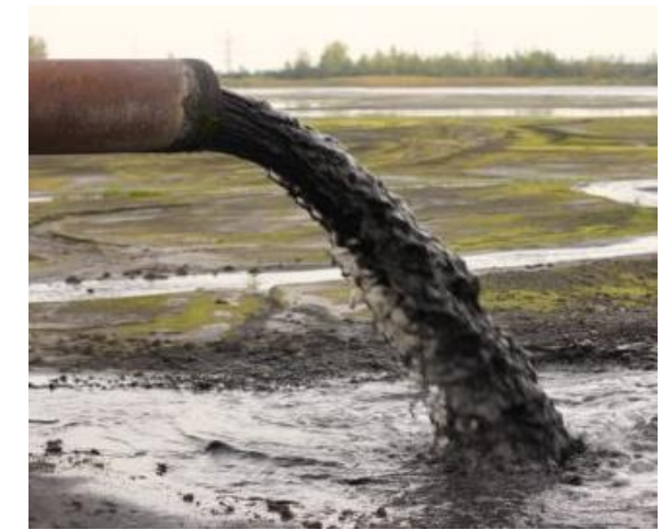
Industrial Effluent Treatment
