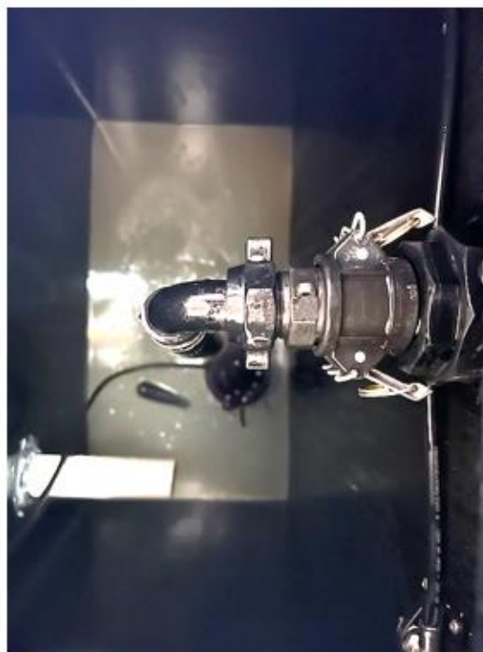
Pump chamber remains clean after 3 months of operation
