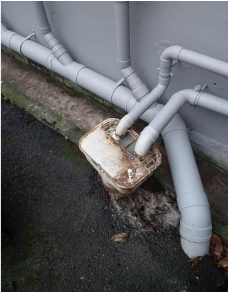
Gully trap overflowing at small café. Grease trap full and no sink screens in use.
